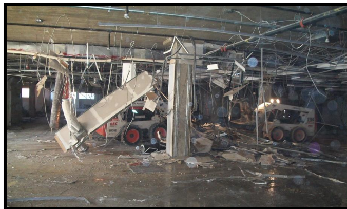
Figure 4: Ceiling Demolition at 7700 Arlington Blvd.
