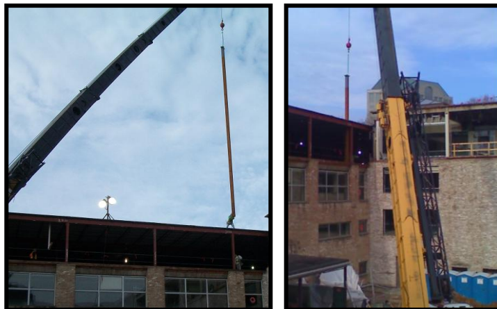
Figure 6: Installation of Progressive Collapse Steel System
