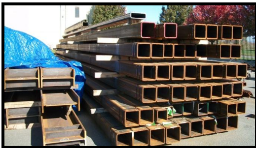
Figure 2: Progressive Collapse Steel System Storage Area
